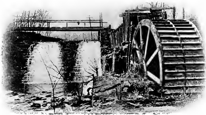
MILL DAM AND WHEEL, GLEN PARK. A LOSS THAT COULD BE RESTORED AND A SKATING POND FORMED. FEW OF THESE OVERSHOT WATER WHEELS ARE LEFT IN THIS COUNTRY.
